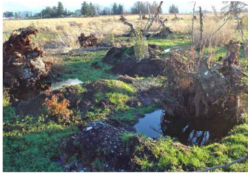
Small pits and mounds were dug by an excavator as it placed large woody debris in this project.
